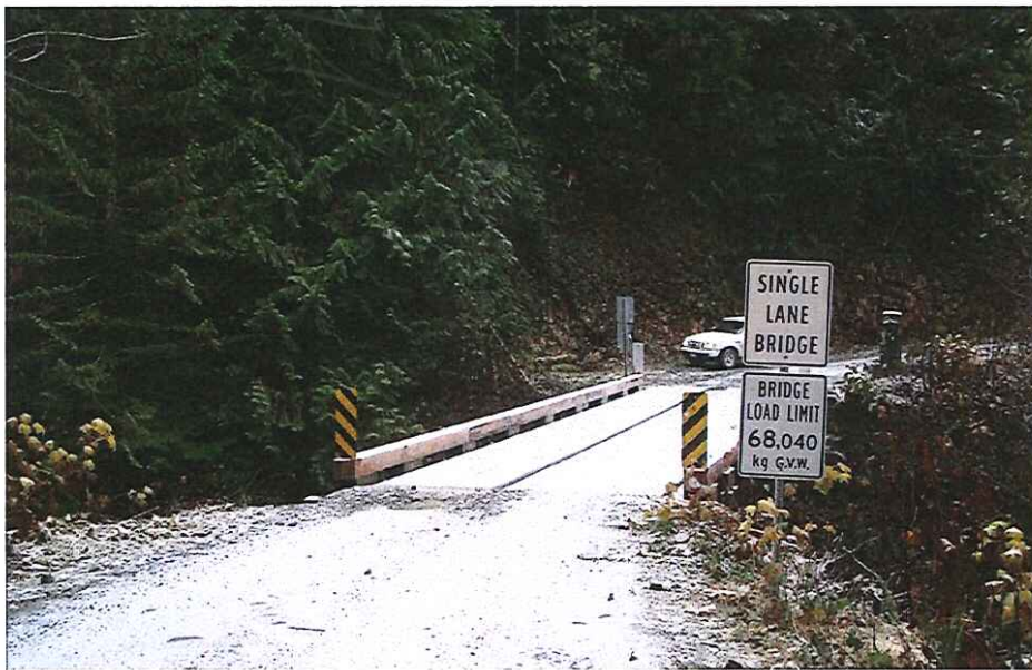
CK2140 Approach Right Bank
