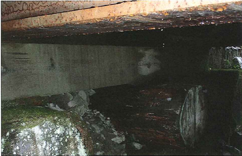
CK2140 Abutment Left Bank
