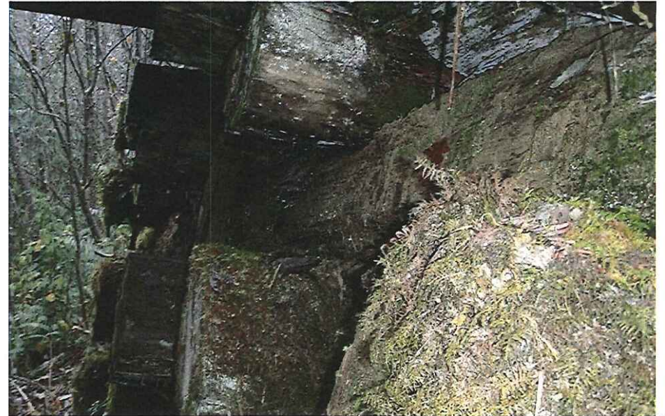
CK2140 Abutment Right Bank #2
