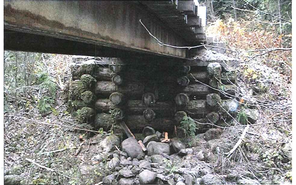
CK2140 Abutment Right Bank
