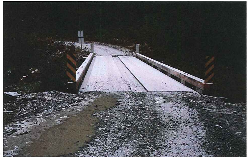
CK2140 Approach Left Bank
